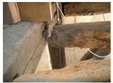
Fig. 1 Detached floor joists
