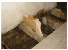
Fig. 6 Header box to assist pouring of TG6
