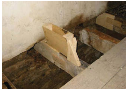
Fig. 6 Header box to assist pouring of TG6
