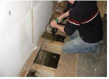
Fig. 3 Slots being drilled into the original floor joists
