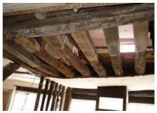
Fig. 6 Underside of the repaired beam prior to being contoured
