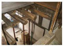
Fig. 2 Propped floor joists with decay removed
