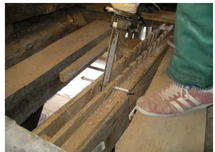
Fig. 3 Slots being cut with a jig and modified chainsaw
